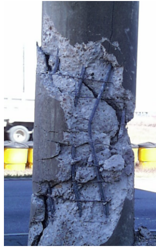
Figur 4: Punching shear feilmodus, (Texas Transportation Institute, 2010)
