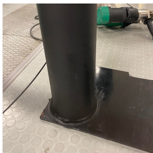
Figure 7.11: Float Top-cap weld
