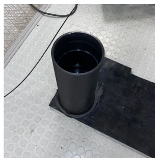
Figure 7.12: Weld water test
