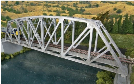
d. Truss bridge
