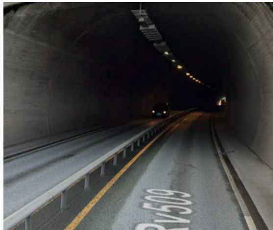
Figure 47: The real Åsnuttunnelen [7]
