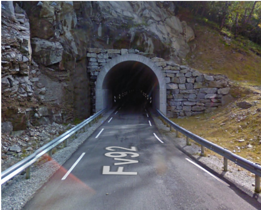
Figure 53: Dørefjelltunnelen with only one driving lane [8]
