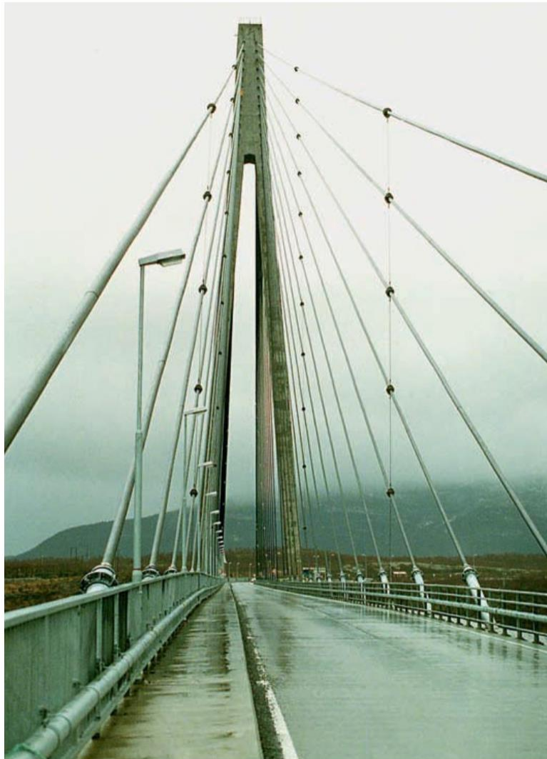
Figure 2.12 Stay cables tie-downs
