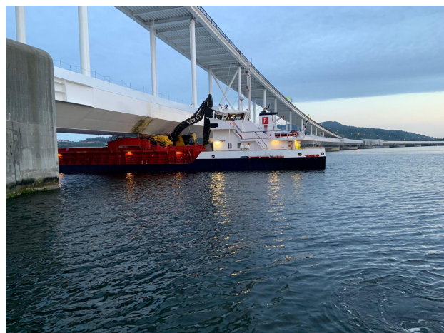
Figure 4.8: Ship Collision at Nordhordland Bridge in 2019 [14]
