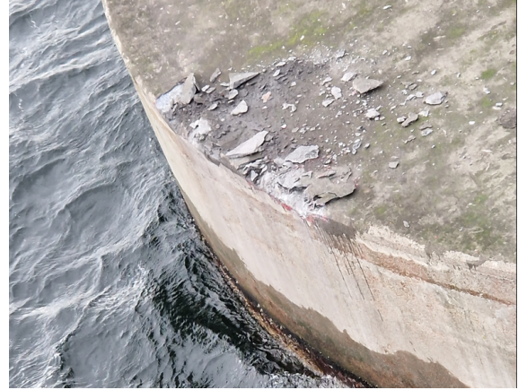
(b) RC pontoon after collision
