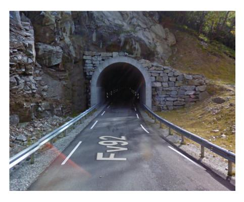
Figure 53: Dørefjelltunnelen with only one driving lane [8]
