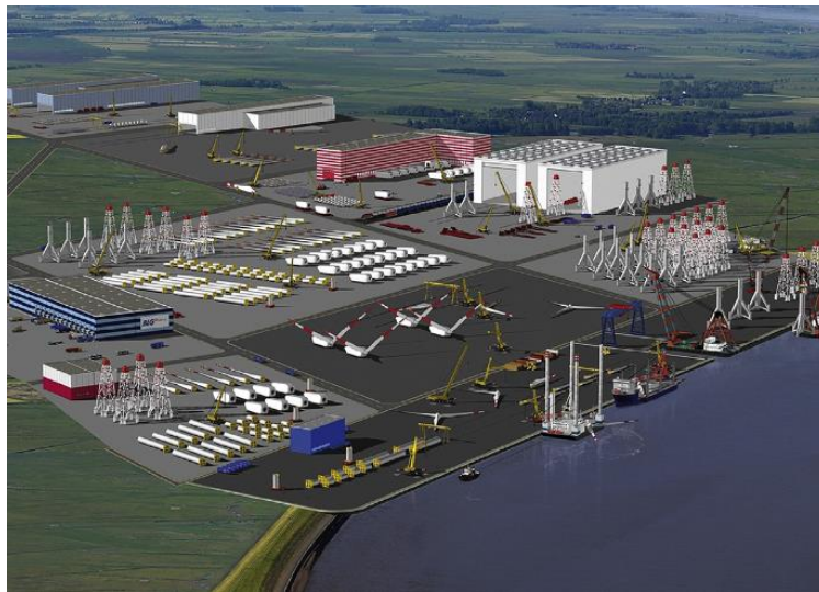
Figure 19. Example of an assembly site [19].
