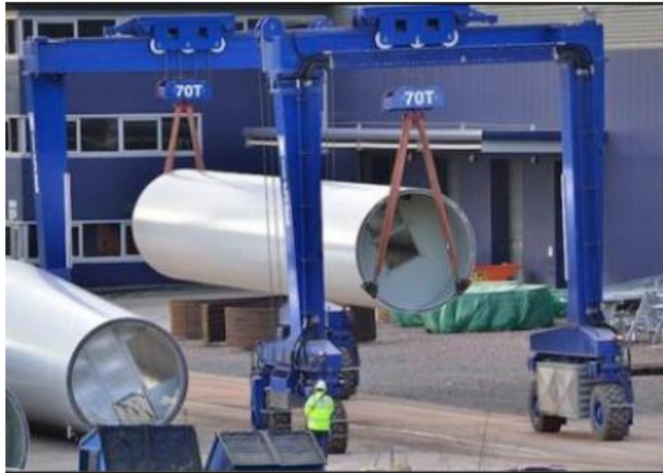
Figure 25. Transport of the tower sections at the port [28].
