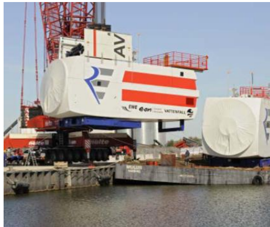
Figure 22. Deployment of the nacelle [28].
