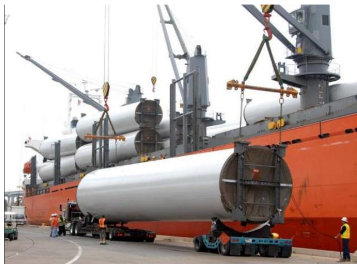
Figure 23. Deployment of the tower sections [28].
