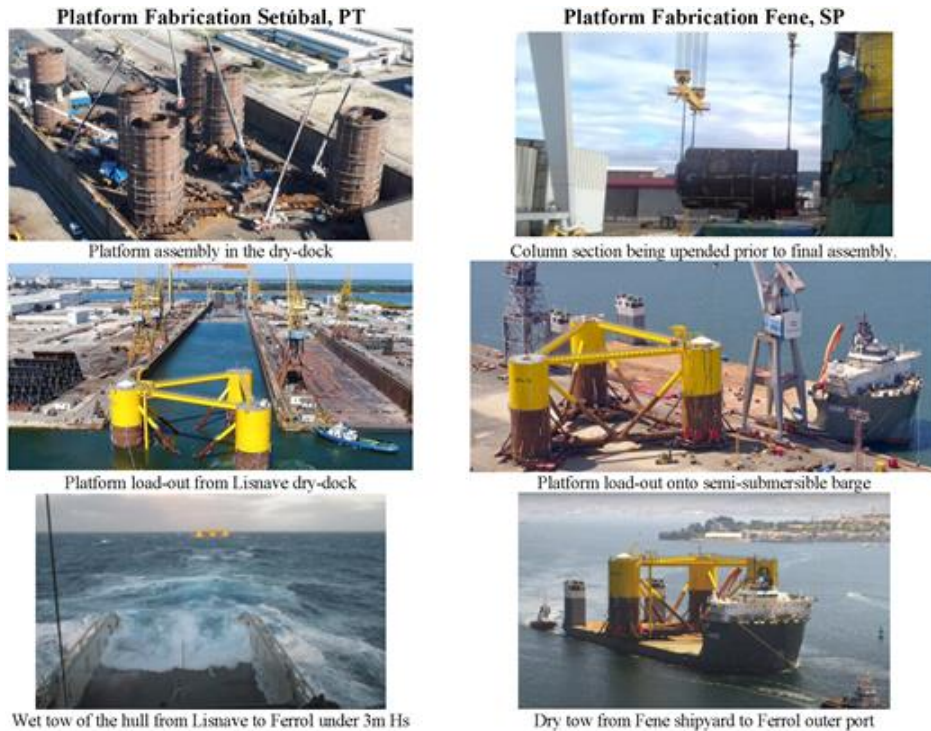
Figure 2.23: Hull assembly in Portugal (left) vs assembly in Spain (right). [2]
