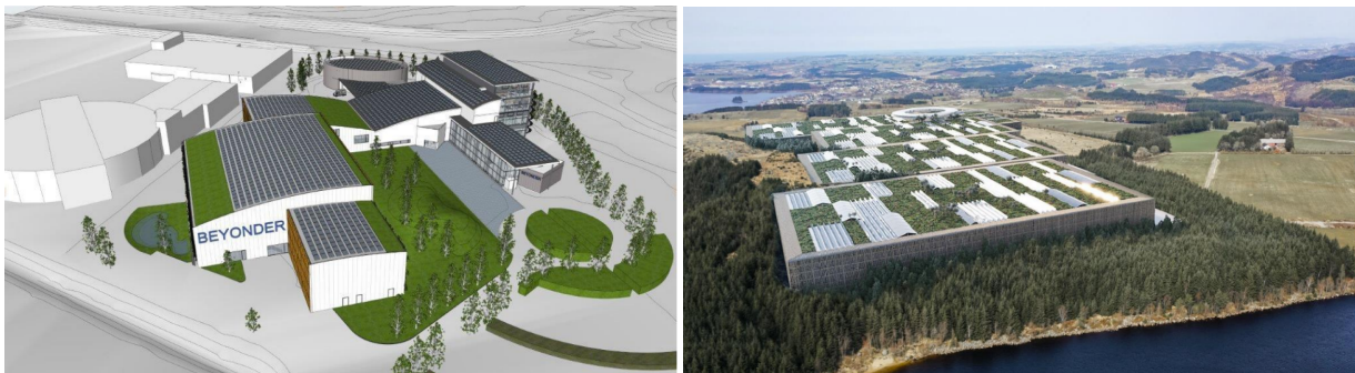
(a) Battery center [Appendix 1, p.10]
