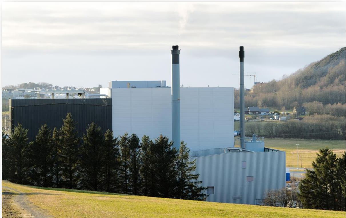
Figure 16 - The incineration plant at Forus.
