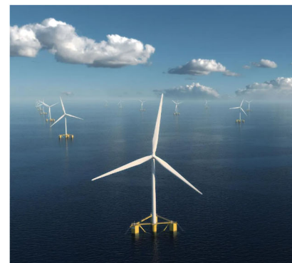
FIGURE 2 Left: DeepCwind semi-submersible floating offshore wind turbine (FOWT) platform 1/50 scale model. 30,32 Right: An example of operating FOWT.
