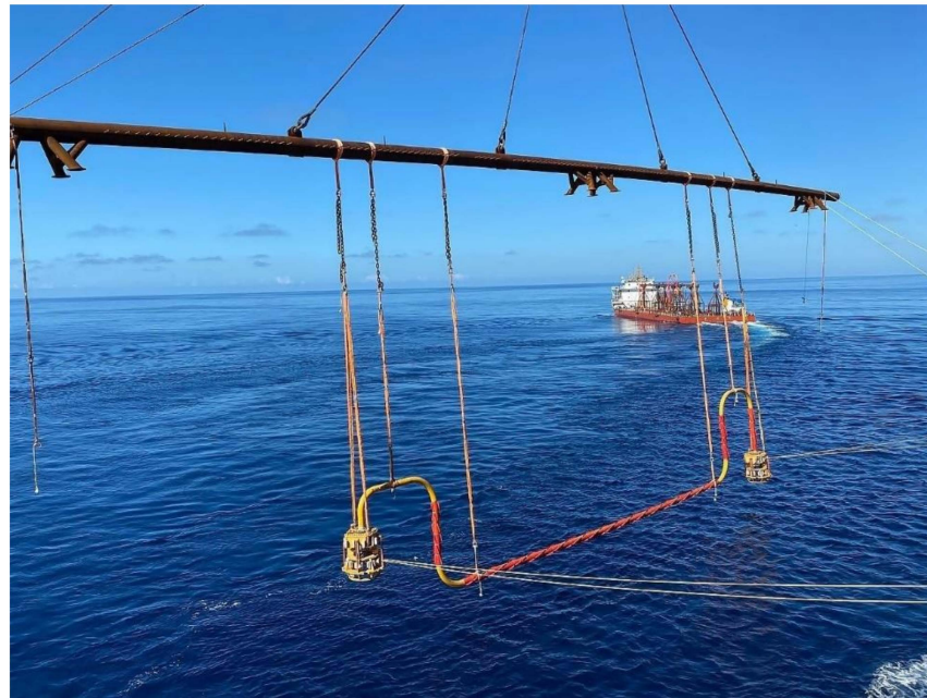
Figure 1. Ready for installation of M-shaped rigid jumper [2].
