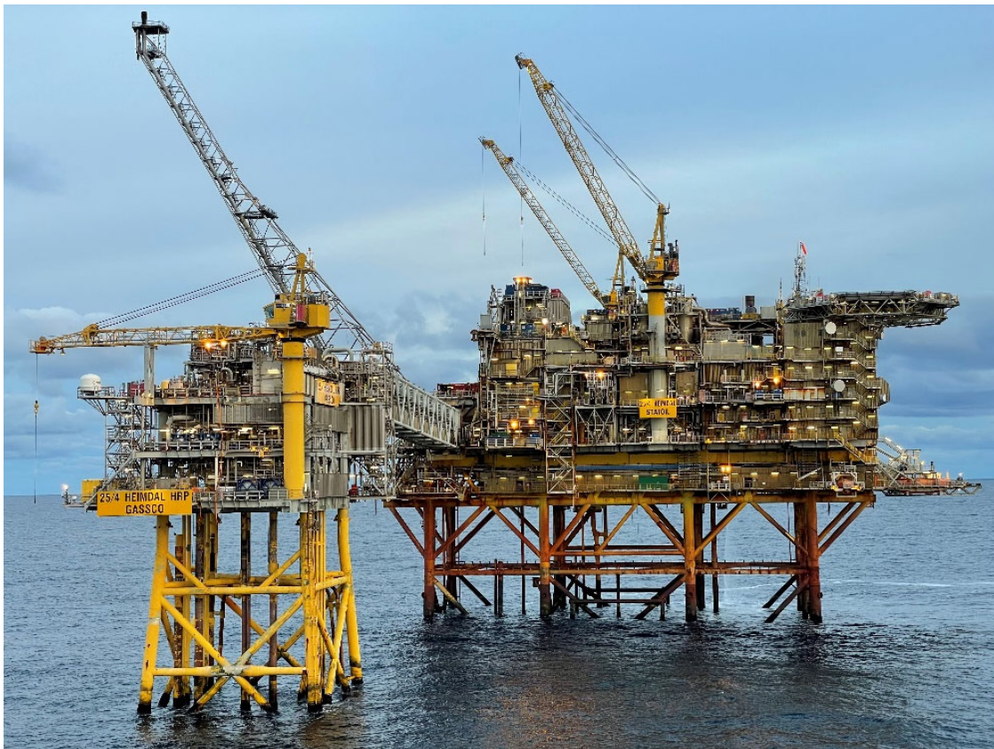
Figure 1. Heimdal platform, typical offshore jacket structure (photo by Simen Riise)
