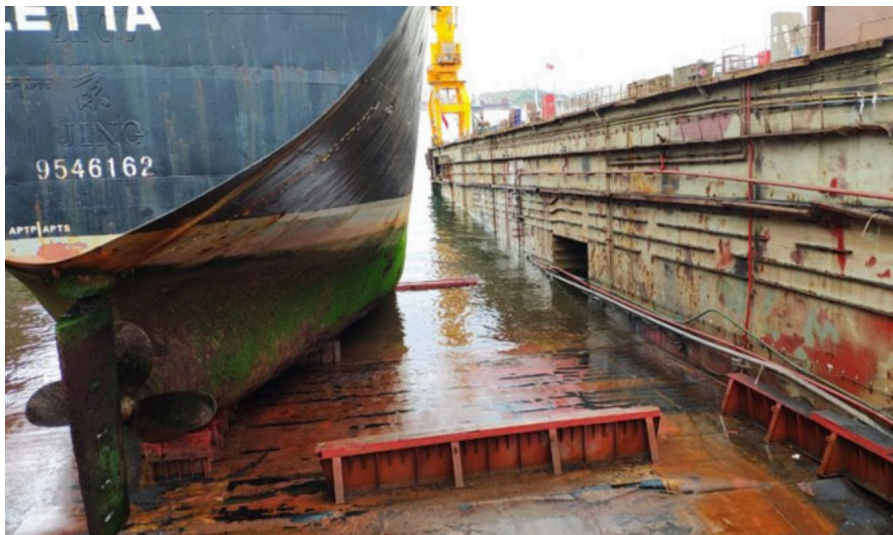
Figure 2. Floating dock in an accidental condition at Tuzla Ship Repair Yard [8].
