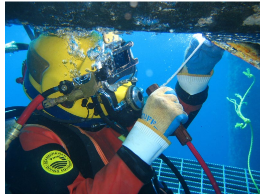
Figure 3-6: Wet welding (AWS, 2017)
