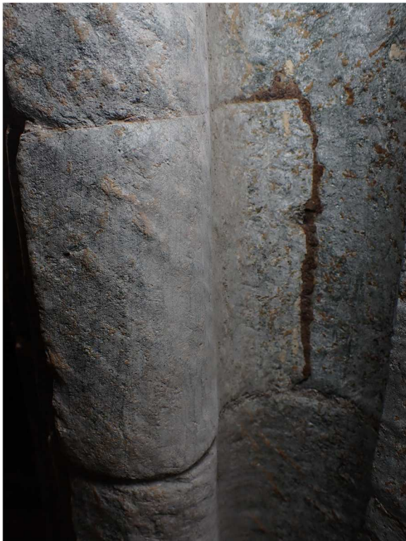
Figure 4. Medieval tar repair on Stavanger cathedral. Image: Museum of Archaeology, University of Stavanger.
