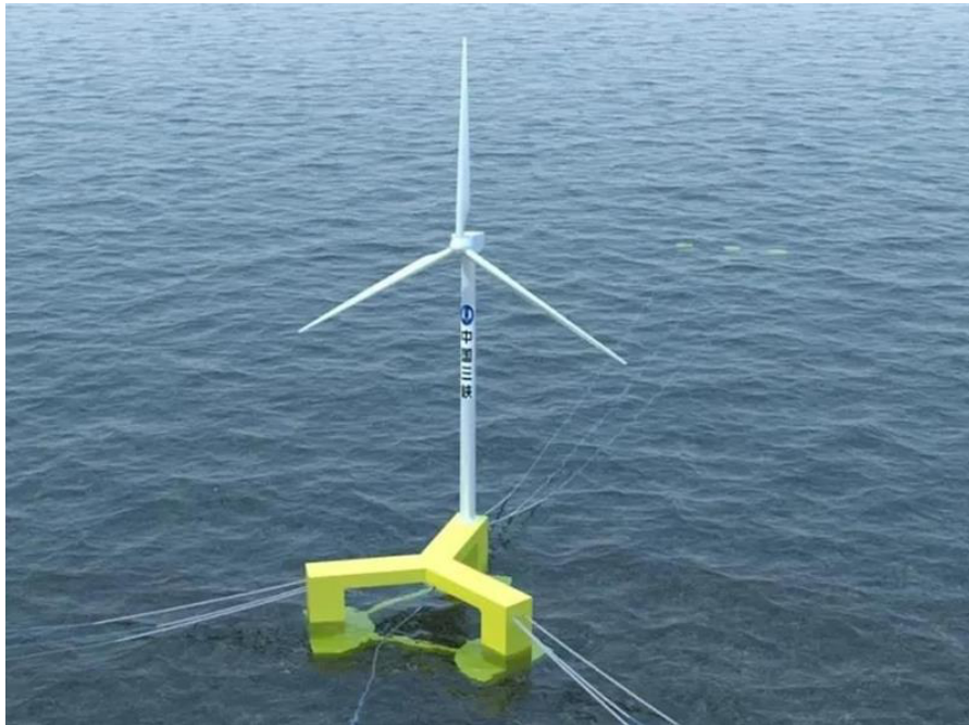
Figure 1. An example of FOWT in offshore field operation.
