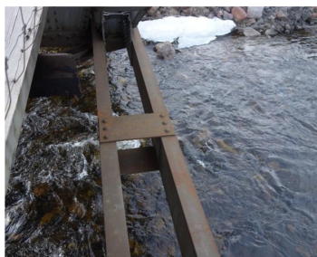
(c) Bottom chord longitudinal beam
