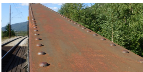
(b) Main truss girder
