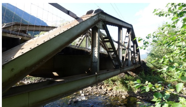
(a) Right side of the bridge
