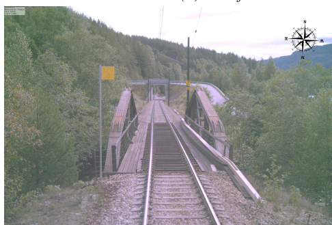
(b) View from the track (view toward the South)
