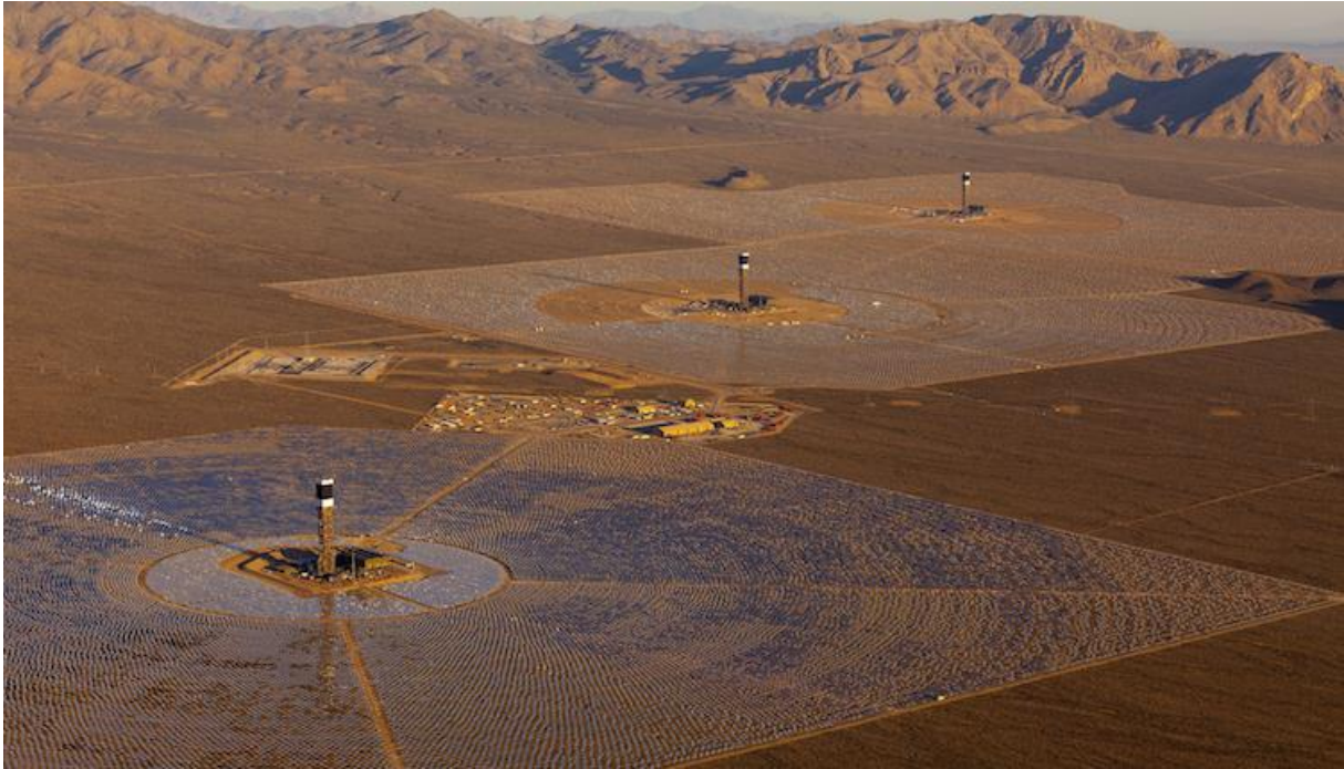
Figure 16. Ivanpah, the largest concentrating solar power installation in the world, was completed in January 2014. The amount of solar thermal energy produced in the US nearly doubled from the previous year. (U.S department of Energy, 2023)
