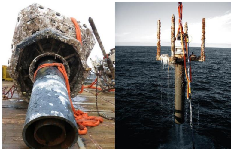
Figure 5-2 Wellhead and multi string conductor removal (www.claxtonengineering.com)
